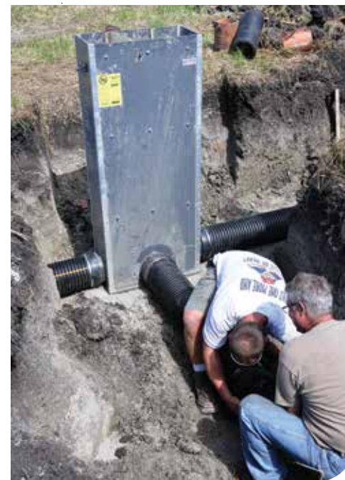
Conservationist Bruce Voigts explains how stop logs slide down into a water control structure to control water levels in a saturated buffer in north central Iowa. Solar powered measuring equipment documents water flow and weather conditions.
